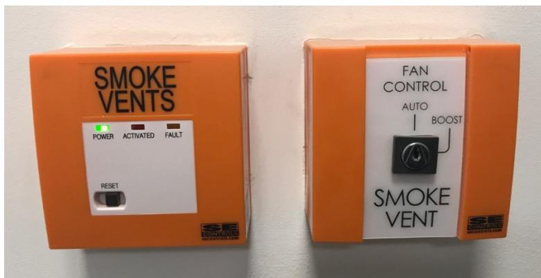
*Figure 2 The design, positioning and precise function of switches can vary greatly from one supplier to another and also from building to building*
